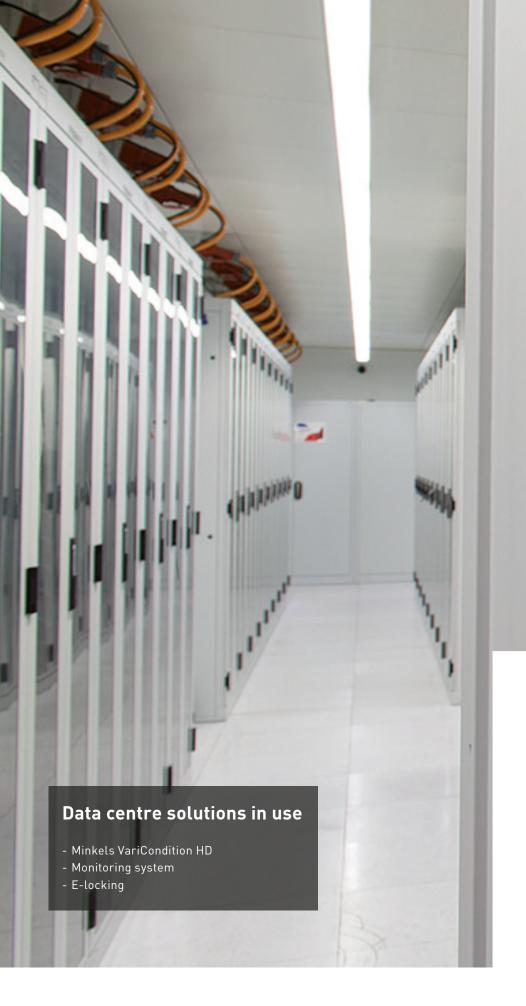
the right places in the rack, ensure a constant climate in the racks and proper management of the cooling system. The temperature difference of 12.5 degrees Celsius between warm and cold airflows provides maximum energy-efficiency in the racks.
