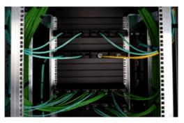
The network is the heart of the IT-infrastructure. Proper cable management provides better performance, serviceability, reliability and airflow management. Using the right accessories for copper and fibre cabling is essential. Especially >CAT 6 copper & fibre is sensitive for sharp bends and minimum bend radius shouldn't be violated. Use modular cable ducts with dividers on top of the rack to manage top of rack cabling smartly.
