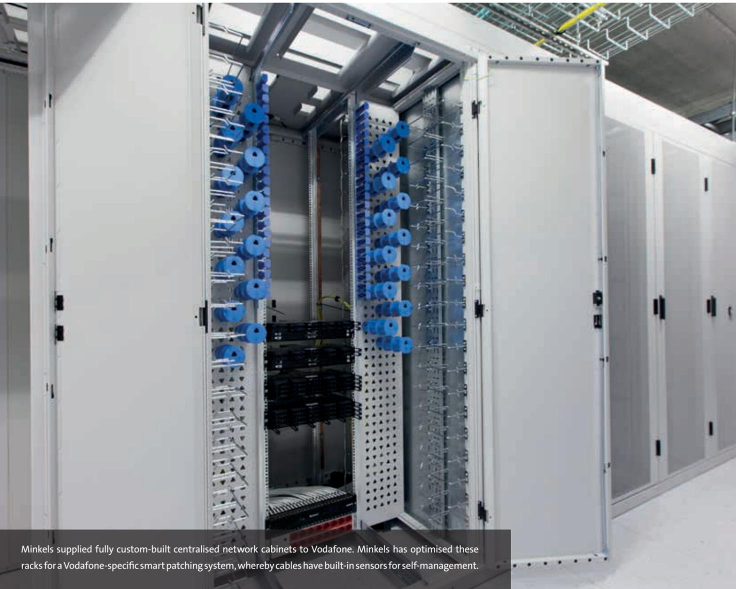
Minkels supplied fully custom-built centralised network cabinets to Vodafone. Minkels has optimised these racks for a Vodafone-specific smart patching system, whereby cables have built-in sensors for self-management.
