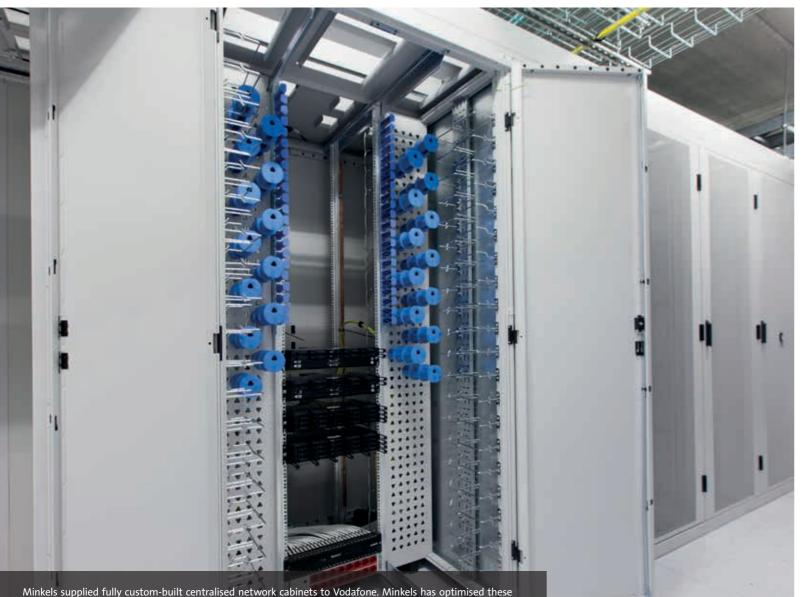
Minkels supplied fully custom-built centralised network cabinets to Vodafone. Minkels has optimised these racks for a Vodafone-specific smart patching system, whereby cables have built-in sensors for self-management.
