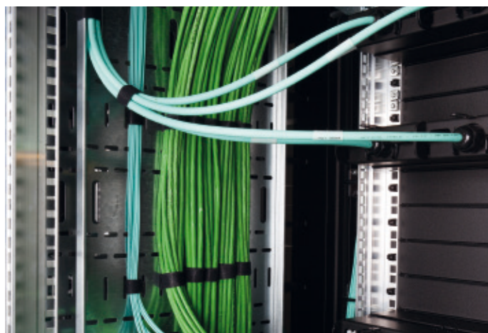
Cable trunking – cables entered from the top
