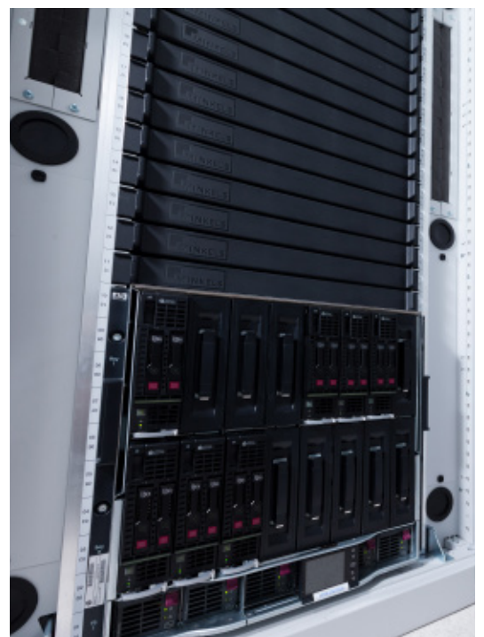
Airtight sealing of a rack
