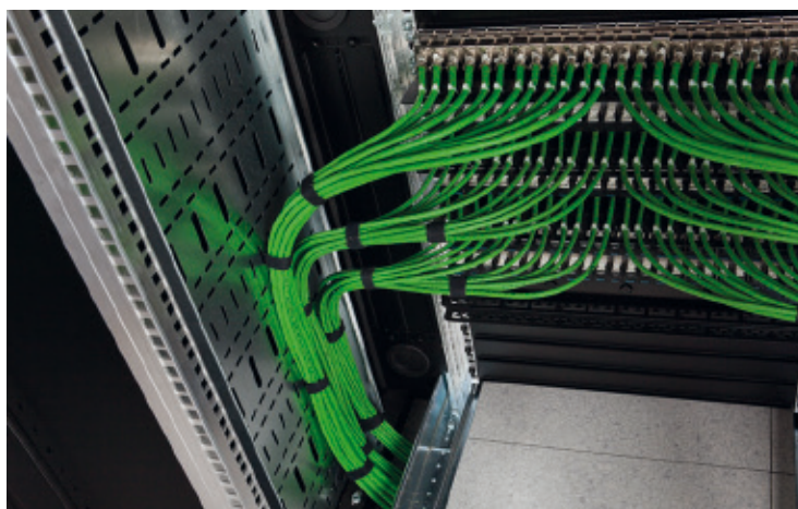
Cable trunking – cables entered from the bottom
