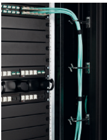
Cable clips on the frame upright
